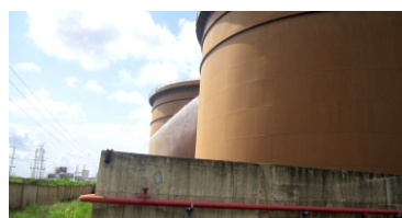
Water being pumped around the tank farm
