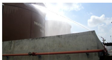
Testing output of firefighting nozzles
